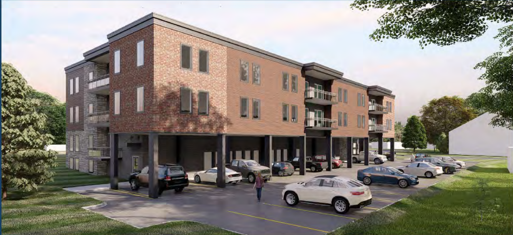
Rear of building, looking south west
