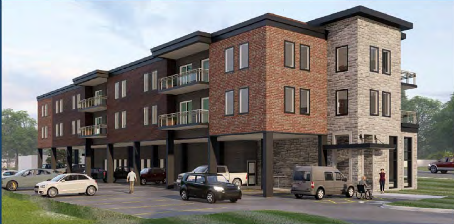
View from Brubacher Street, looking south east (rear of building)
